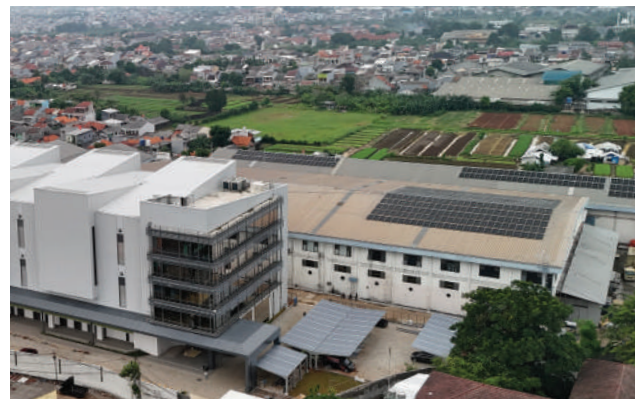
● Panel surya atap on grid di Pabrik Tangerang
